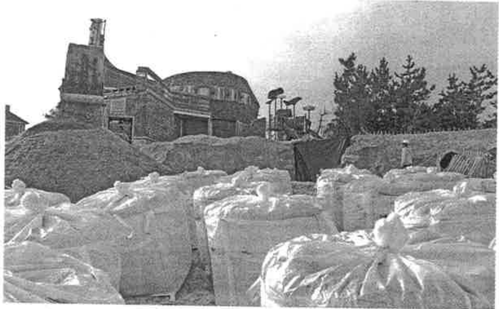
Geocubes were installed at the Quogue Village Beach in 2010.
